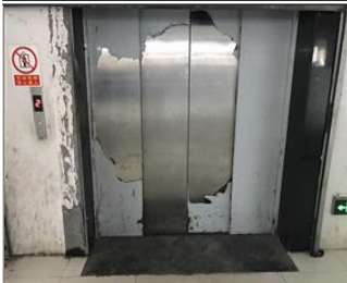
Photo of the inside of the main production hall 2 Elevator.jpeg
