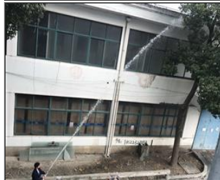
Photo of fire safety equipment 2 Fire hydrant testing.jpeg
